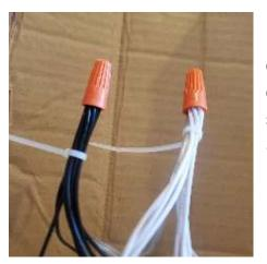
f) For the final part of this step, take your orange plastic wire nuts and screw them onto the ends of each bundle of wires. Be sure to do this in a clockwise direction. Screw on until snug, but not overly tight.
