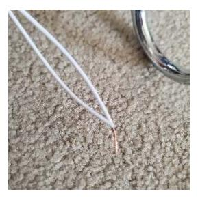
a) Now that all the arms are on your chandelier you should notice each arm has 1 white wire and 1 black. You need to make pairs of the same coloured wires, like shown in the photo on the left. To do this take the exposed wire ends and twist them together in a clockwise direction.
